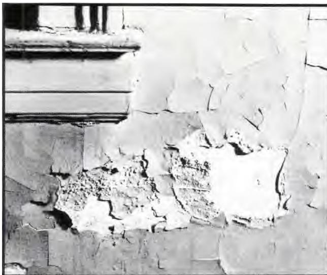
Paint and plaster failure from water penetration.
