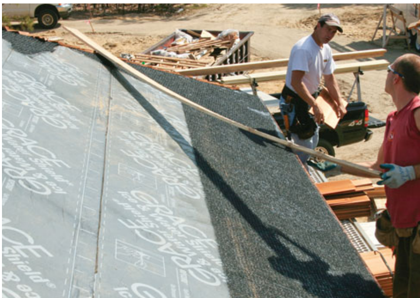
Figure 5. Ventilating Cedar Breather mat installs quickly and provides critical air circulation under the shingles.
