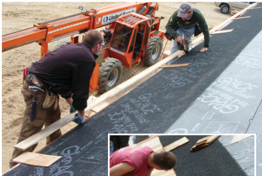
Figure 7. To start the first course, the crew nails a guide strip to a chalk line snapped at the 1½-inch overhang (above). Fence boards ripped to the exposure width guide the successive courses (right).
