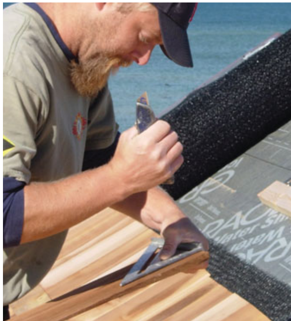
Figure 3. The straight grain of a premium-grade cedar shingle slices cleanly with a utility blade. Excessively wavy grain can contribute to cupping or warping.
