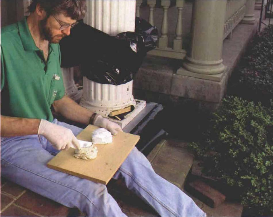
**Two-part fillers are mixed on a board.** After measuring the right amount of resin and hardener paste, the two are kneaded together on a scrap of plywood.
