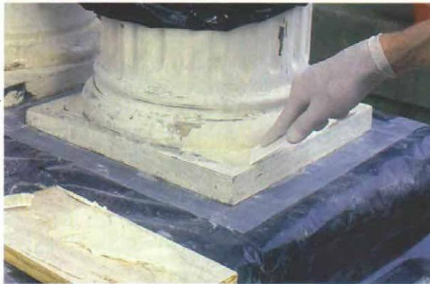
**Primer protects the epoxy.** As a final step before painting, a coat of primer is applied to seal the repair against moisture as well as against UV-radiation, which can damage some epoxies.
