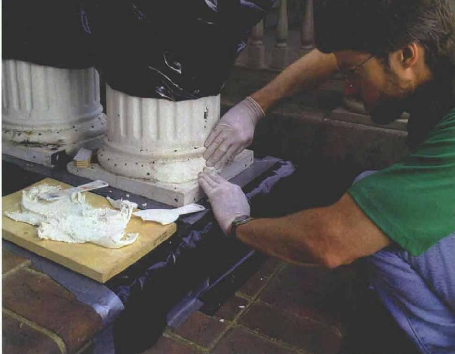
**The rest of the hole is filled by hand.** Epoxy paste is packed into the repair by hand until the entire gap is filled.
