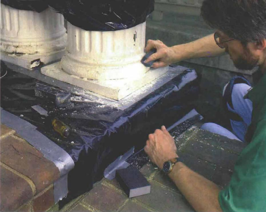
**Woodworking tools also handle epoxy.** Cured epoxy can be worked like wood. A chisel and a Surform plane rough out the shape, and sandpaper does the smoothing.
