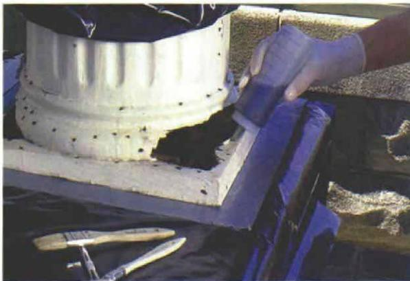
**Consolidant is injected into the repair.** Liquid epoxy, or consolidant, is squeezed into holes drilled around the repair. The consolidant saturates the soft wood, making it rock hard.
