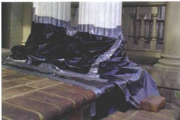
**All dressed up.** The same poly tent that is used to keep moisture away from the repair while it dries also protects the epoxy from weather while it cures.
