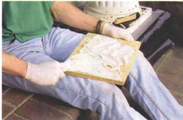
**Wood blocks save on epoxy.** To keep from using large quantities of expensive epoxy, blocks of wood are encapsulated in the epoxy to act as aggregate.
