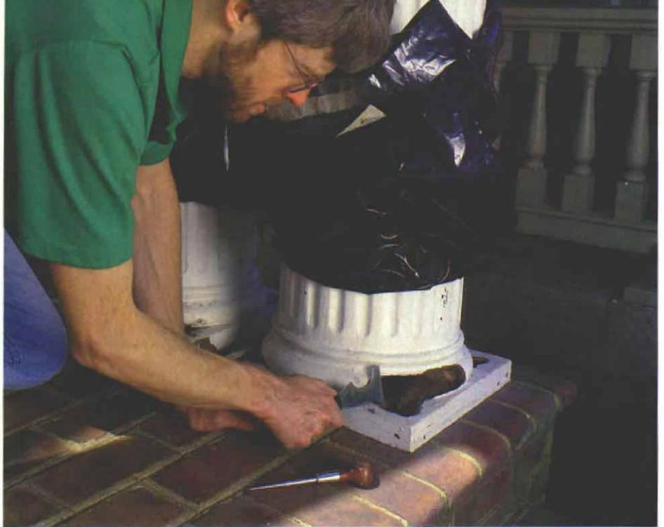
**Getting down to sound wood.** The first step is removing loose, crumbly wood. A five-in-one painter's tool and an awl are best for digging out any wood that is not still firmly attached.
