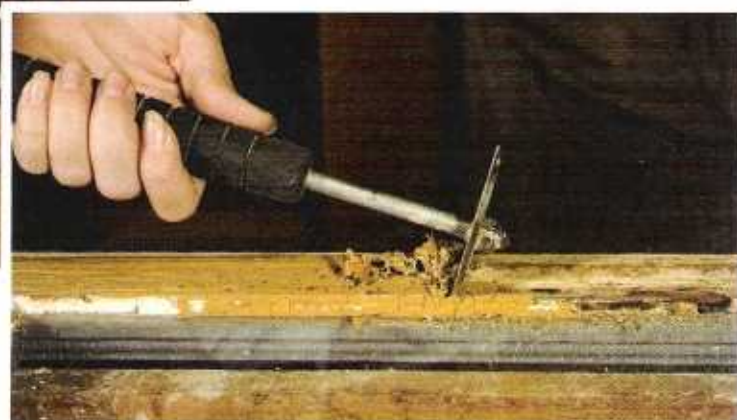
Figure 2. Placed over a heat shield to protect the glass, an infrared paint remover softens up the glazing compound and paint (left). After a minute or so, both materials release their grip on the wood and can be quickly scraped off (below). A special chisel with an adjustable guide wheel removes glazing compound without harming the glass (bottom).
