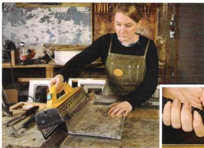
Figure 2. Placed over a heat shield to protect the glass, an infrared paint remover softens up the glazing compound and paint (left). After a minute or so, both materials release their grip on the wood and can be quickly scraped off (below). A special chisel with an adjustable guide wheel removes glazing compound without harming the glass (bottom).
