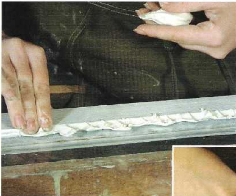
Figure 3. Holding a ball of glazing putty in one hand, a worker tears off manageable chunks and presses them in place with her fingers (above). When one side of the sash is fully loaded, she tools the compound smooth with a glazier's curved putty knife (right).
