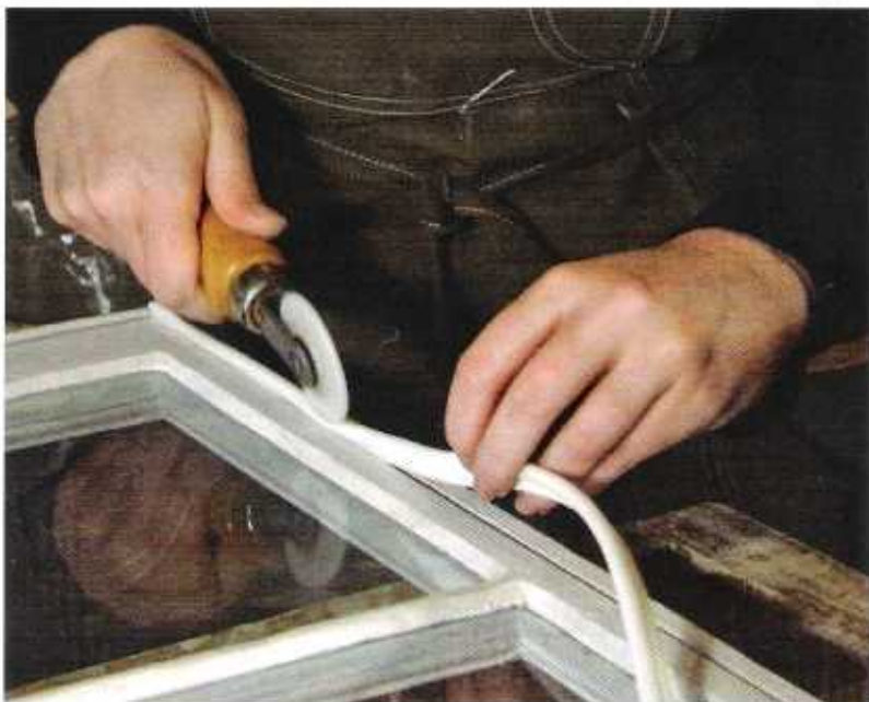
Figure 4. The author prepares a sash to receive weather stripping by routing a 3mm groove into the mating surfaces of the sashes (top). After the sash is fully primed, horizontal surfaces — such as the meeting rail shown above — are fitted with silicone bead. On the exterior of each sash, vertical surfaces are fitted with brush-type weather seals, which seal tightly to the stops but don't interfere with opening and closing.
