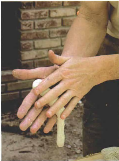
A putty rope is easier to work into the frame. Roll the putty between your hands, and use your fingers to press it into the sash.
