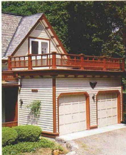
and ensured positive alignment of the vertical members. The tops of the partial balusters are housed completely in the groove, but the tops of the full-length balusters also have stub-tenons, cut on the radial-arm saw.
