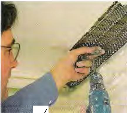
Expanded metal mesh is the modern lath common since the 1920s and widely used for large repairs. Here, a piece is cut to the patch shape and screwed right over the old wood lath to improve anchoring for the plaster scratch coat.
