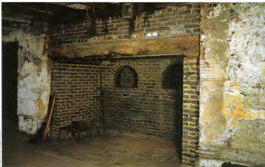
Prior to the late 19th century, plaster was a mixture of aggregate (usually sand), fiber (such as animal hair), water, and lime that set slowly but could last for centuries, as in this mid-17th century house in Massachusetts. The lime came from heating and grinding limestone or oyster shells, bits of which sometimes appear in the undercoats. Gypsum became a common plaster ingredient by 1900 because it set quickly.
