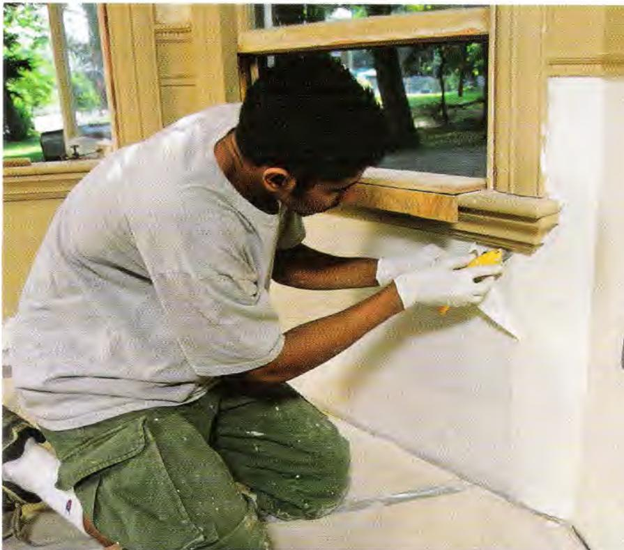
Though cotton textiles can still be found, most of the liners used for wall canvassing today are manmade fiber products ordered through wallpaper stores. Though they can't bridge holes or disguise uneven patches, they are a user-friendly way to resurface and preserve basically intact plaster.
