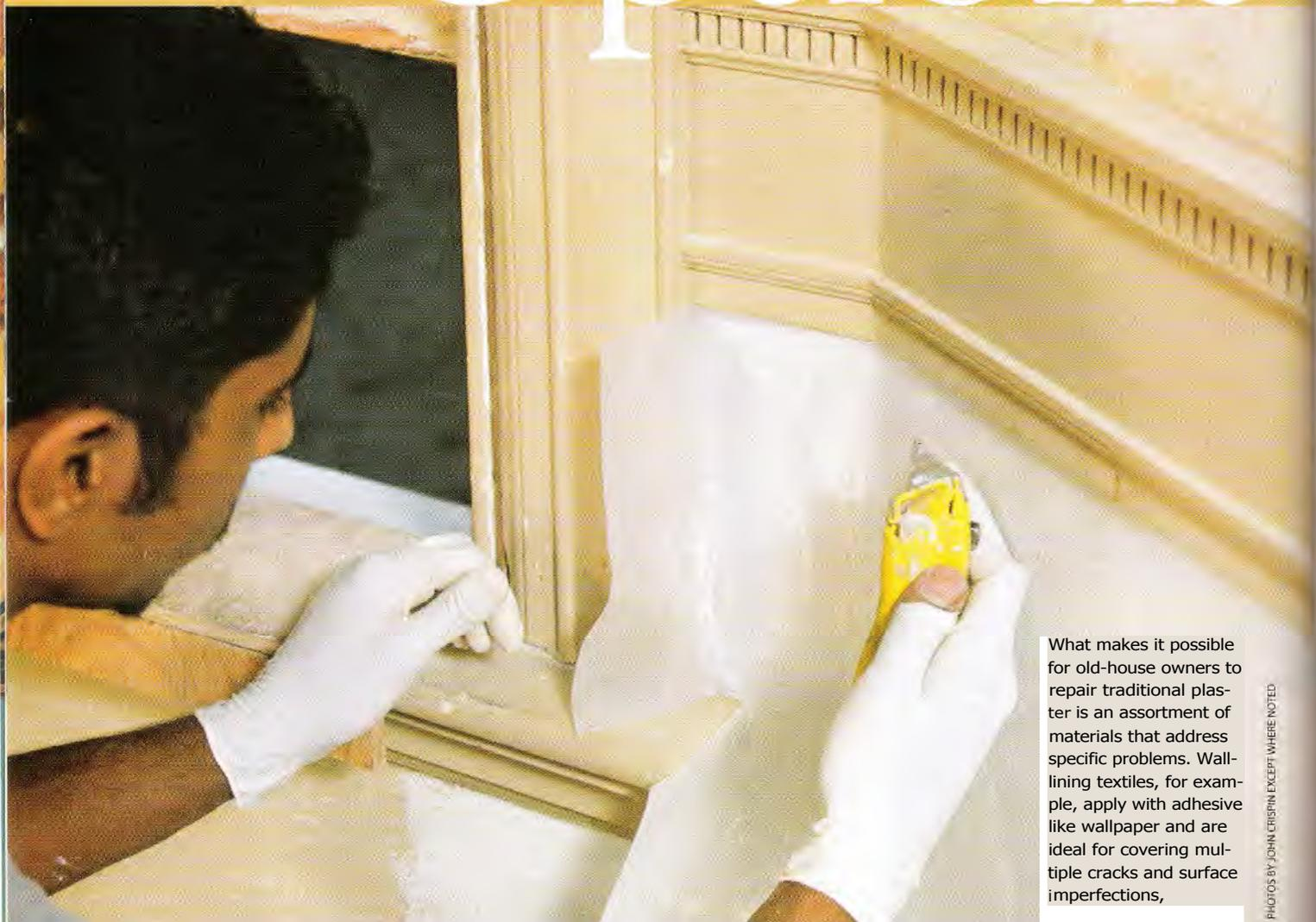
What makes it possible for old-house owners to repair traditional plaster is an assortment of materials that address specific problems. Wall-lining textiles, for example, apply with adhesive like wallpaper and are ideal for covering multiple cracks and surface imperfections,
