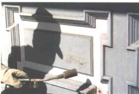
Using a propane torch, a painter heats the old paint until it blisters (above). Using a scraper, he pulls the softened paint off the wall (below).
