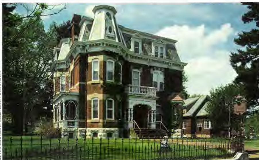
Typical of large, three-storey mansard houses in the Midwest is this example in Jefferson City, Missouri. A prominent two-storey bay window on the left is topped by a stub mansard tower, while the right corner features an unusual first-floor bay set on the diagonal.
