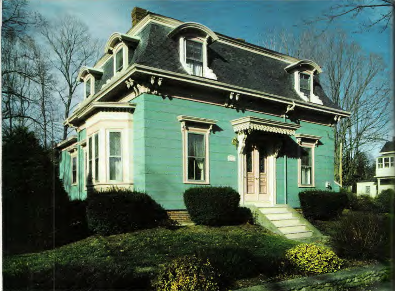
One-storey mansard houses pop up periodically, but certainly not in large numbers. This Topsfield, Massachusetts, house with a concave curved roof retains the usual dormers, a fine left-side bay window, and a distinctive console hood over the double front door.
