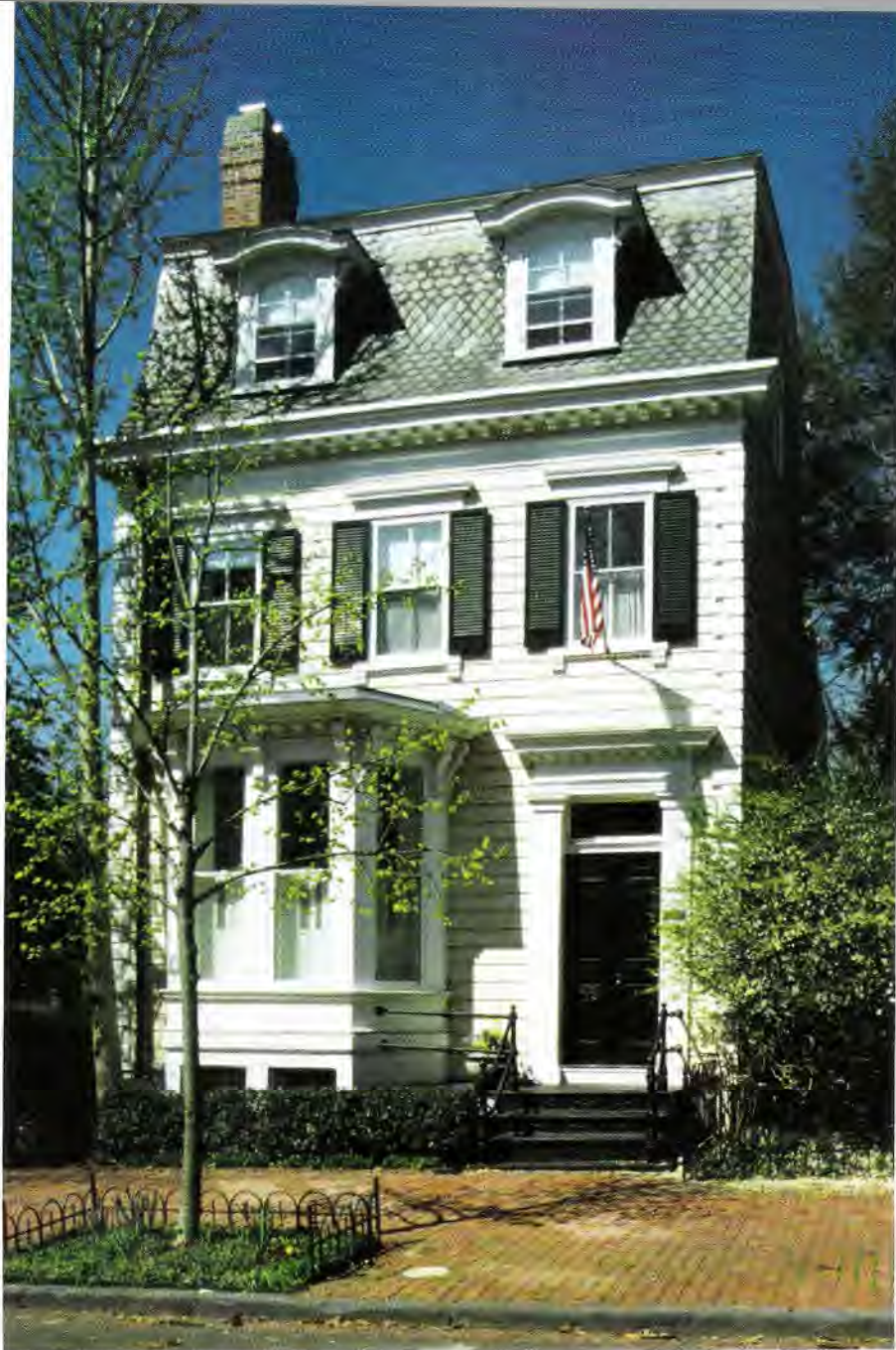
This modest-frame Second Empire house in the Georgetown Historic District of Washington, DC, carries the style in simplified form. The bay window, door, frontispiece, corner quoins, and modillion cornice provide a comfortable degree of ornament for a smaller residence.
