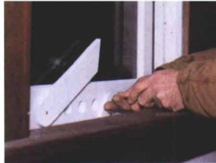
**A compound angle ensures a tight fit.** Shaped from an 11 in. piece of poplar and cut at a compound angle, the small end of the vent-hole cover is secured with two screws to the inside of the storm window.
