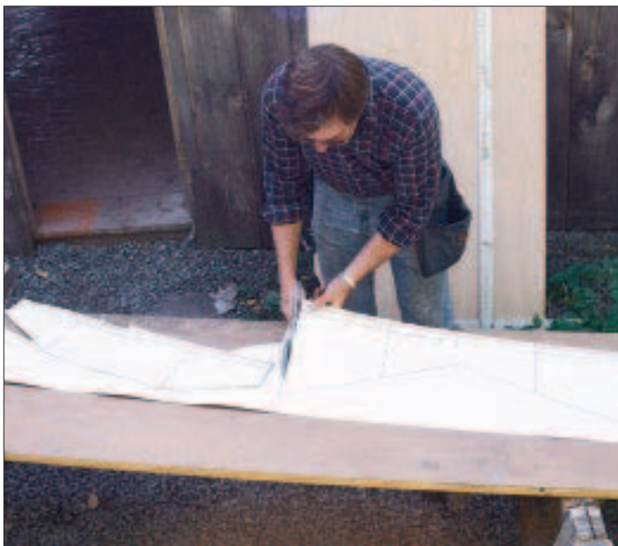
Figure 3. The author cuts the upper and lower pieces of counterflashing from painted-aluminum coil stock (.019 inches thick). The tapered cuts match the roof pitch; layout lines mark the folds at the chimney corners.
