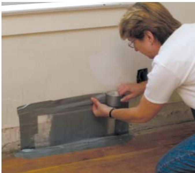
**Figure 1.** Sealing off this cold-air return duct ensures that job-site dust does not get blown throughout the house.
