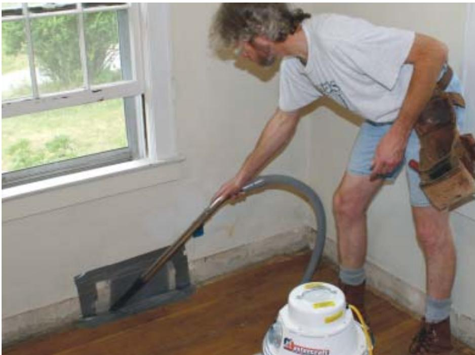
**Figure 4.** After the dirty work is done, all surfaces and crevices should be slowly and thoroughly vacuumed with a HEPA vac.
