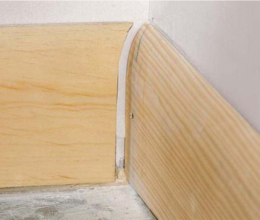
**W**hen two pieces of trim meet at an inside corner, you could miter the joint, but most professional carpenters prefer to cope. An airtight coped joint is easier to produce: It doesn't require the perfectly square corner that a mitered joint needs. A coped joint is also less likely to open up after a few seasons of expansion and contraction.
