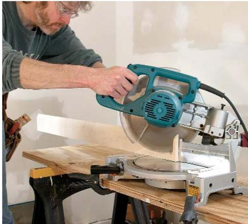
**1** **Miter cut determines the profile.** Although you can trace the profile from one piece of trim to the other, a 45° inside miter cut achieves the same purpose. An efficient carpenter chops all the profiles for a particular room at the same time, then cuts each piece of trim to length later.
