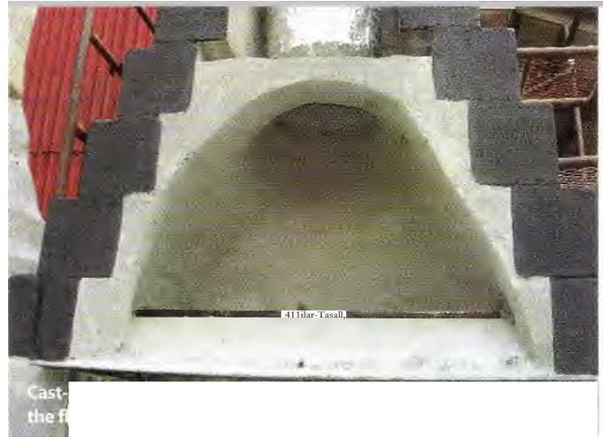
If the problem chimney has one or more clay flues within it, the installer will determine whether the tile can be left in place or needs to be removed. Determining factors include the structural condition of the existing flue and chimney, and how much space is needed based on the size and number of flues required.
