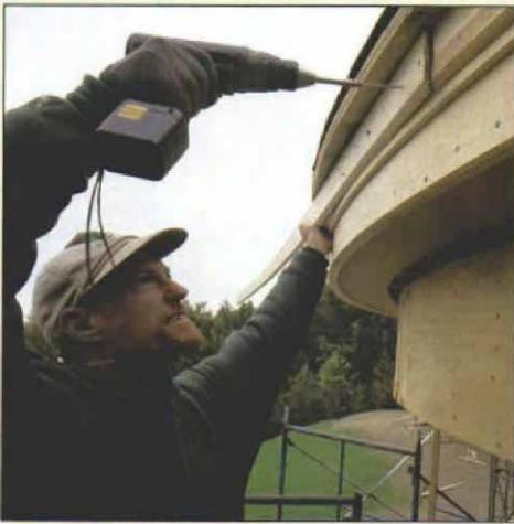
**Layers of trim are built up under the drip edge. To bend the trim around the radius, the crown molding was ripped into pliable strips, then applied in sequence to the outside frieze board. Tight nailing patterns and staggered end joints kept the curves fair.**
