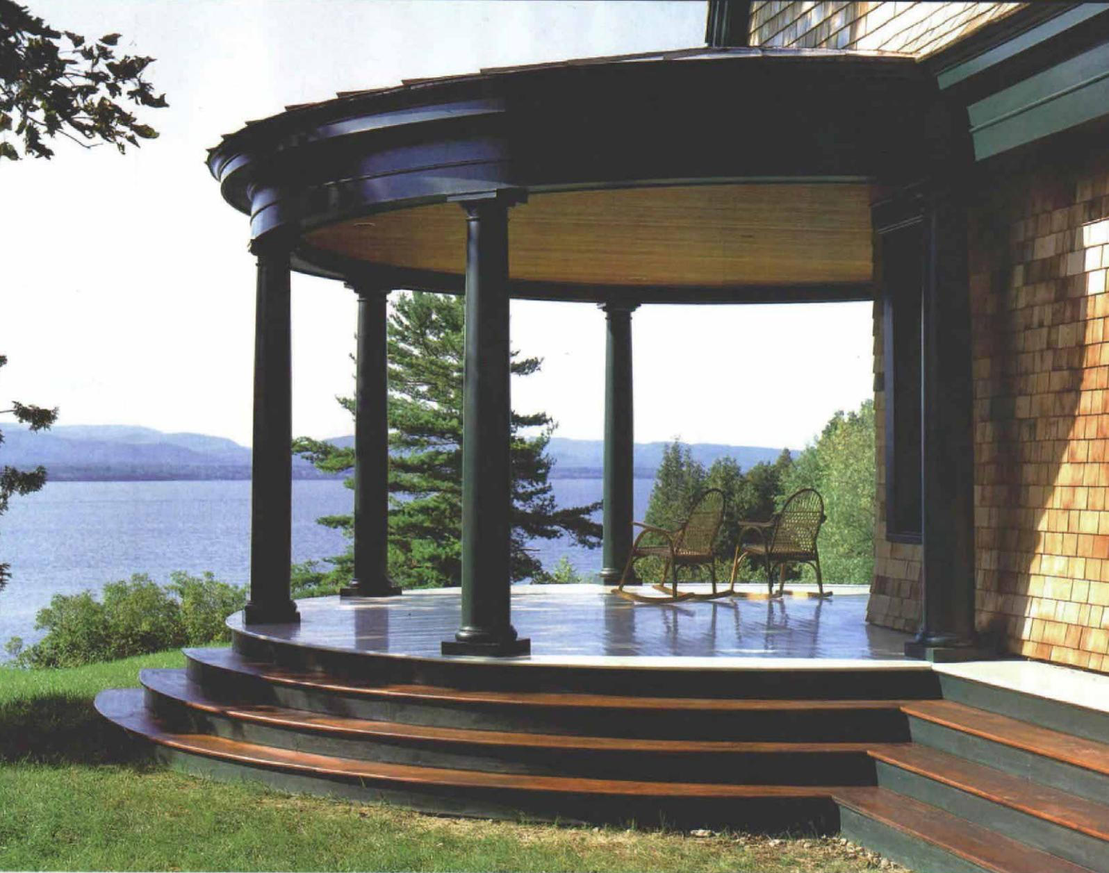
**A few strategically placed columns support the roof.** Because the weight of the roof was evenly distributed on the rigid laminated beam, columns were required only beneath the section joints. The resulting open spans also give room to enjoy the view.
