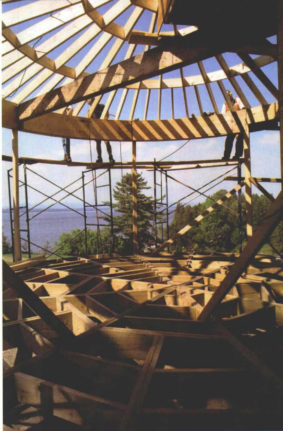
**Building in the round relies on the art of framing.** The floor frame slopes from a central point to shed water and was configured to support a radial pattern of decking. Consistent spans between the rafters above meant plenty of support for the roof sheathing.
