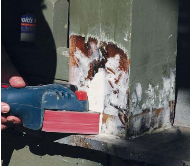
Figure 5. Specialty sanders, like this Bosch compact belt sander (above), are indispensable for finishing an epoxy patch. For paint-grade work, a random orbit sander loaded with 100-grit paper makes the patch disappear (right). No repair is complete until both the epoxy and the bare wood surfaces are sealed with a premium epoxy-compatible primer, followed by two coats of top-quality acrylic paint (below).
