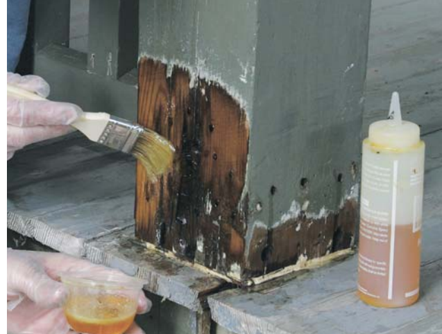
Figure 3. Drilling a series of small holes around the perimeter of a rot-damaged crevice (left) makes it possible to inject epoxy consolidant deep into the wood. To fully saturate the damaged area, the author alternates between squirting consolidant into the holes and brushing it on the surface (below).
