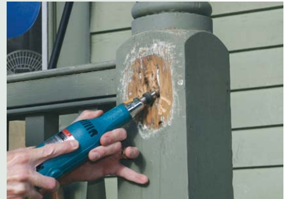
An alternative to fortifying rot-softened wood fibers with an epoxy consolidant is to remove all of the suspect material with a power tool — such as the die grinder shown here, which is equipped with a 1/2-inch-diameter core box bit.
