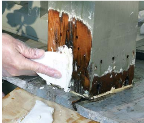
Figure 4. Using a plastic putty knife, the author presses the epoxy paste firmly into the crevice, then wipes the surface smooth (left). After the epoxy has fully cured, he begins the tooling process by shaving down the rough spots with a Surform plane (below).
