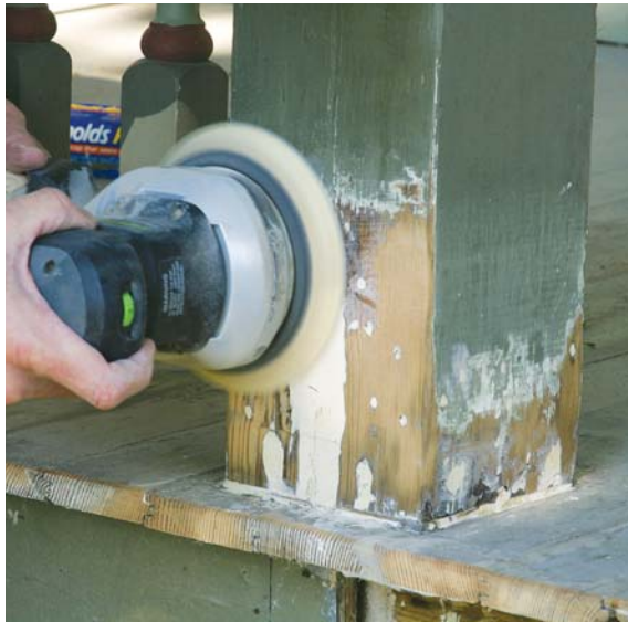
Figure 5. Specialty sanders, like this Bosch compact belt sander (above), are indispensable for finishing an epoxy patch. For paint-grade work, a random orbit sander loaded with 100-grit paper makes the patch disappear (right). No repair is complete until both the epoxy and the bare wood surfaces are sealed with a premium epoxy-compatible primer, followed by two coats of top-quality acrylic paint (below).
