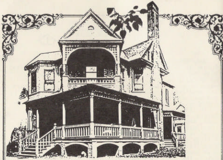
NEIGHBORHOOD HOUSING SERVICES 326 EAST CHICAGO STREET
